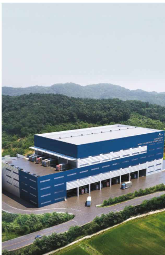
Logiport West Anseong-II, Anseong-si, South Korea
