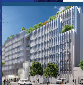
Office development on rue Jeanne d'Arc in Paris
